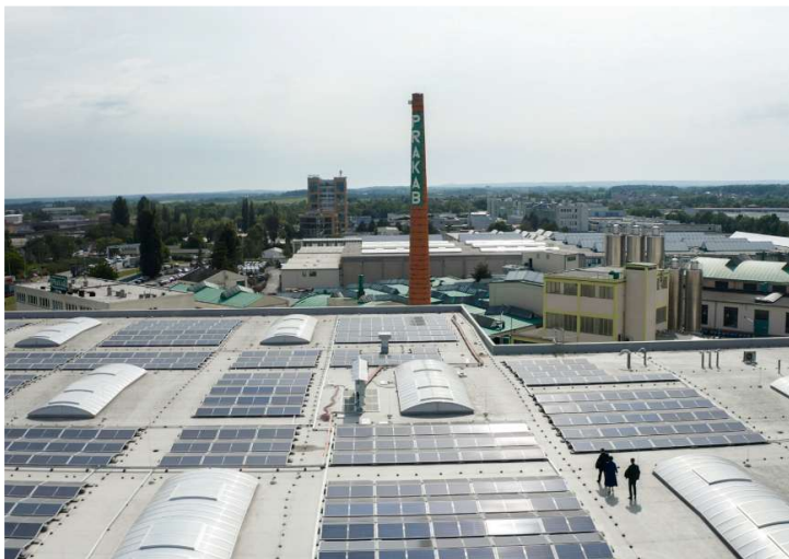
Photovoltaics in Prakab
