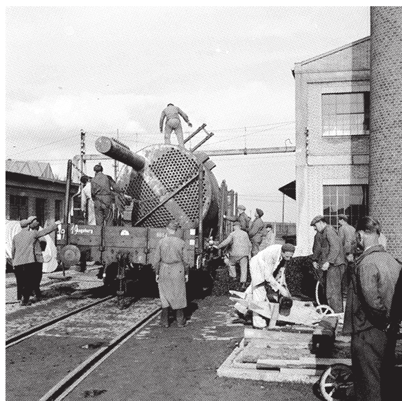
New boiler installation
