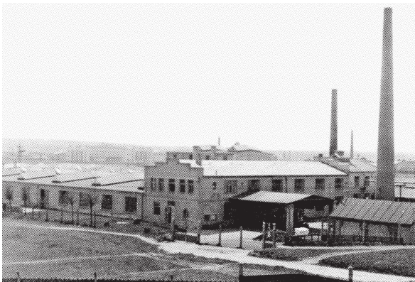
The oldest known image of the factory with the main hall still standing, approx. 1922
