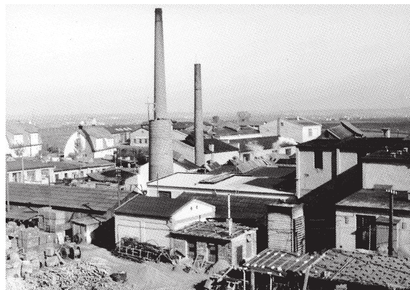
The factory with unfinished chimney, 1940
