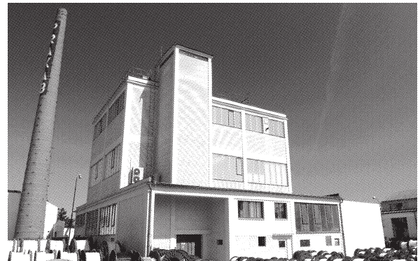
Some of the first flame retardant cables in the world were manufactured here
